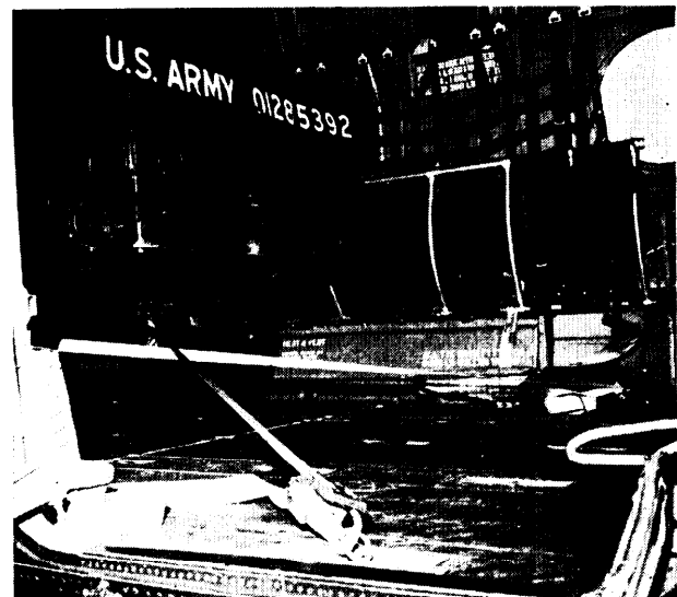
Figure 1. Typical tiedown of M100 1/4-ton trailer. (View through main cabin entrance door.)
